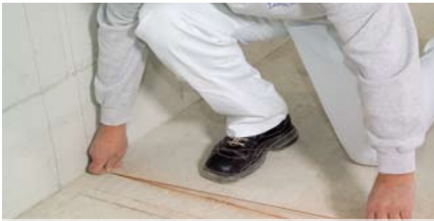
1. Mark partition wall position using a chalk line
