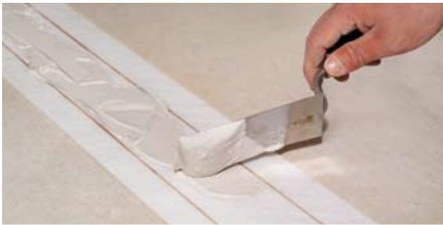
3. Apply gypsum adhesive bed
