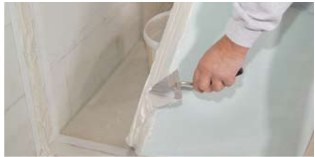
4. Apply gypsum adhesive to the face of the gypsum block and work force-fit
